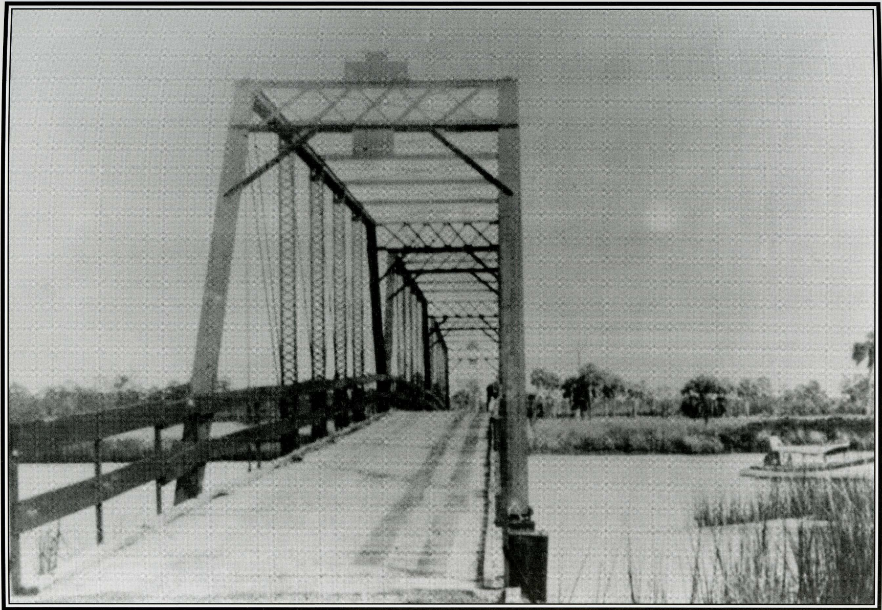
A wooden country bridge crossed Shell Creek near Punta Gorda in Charlotte County from 1915 to 1920. Today, U.S. Highway 17 spans the waterway.
