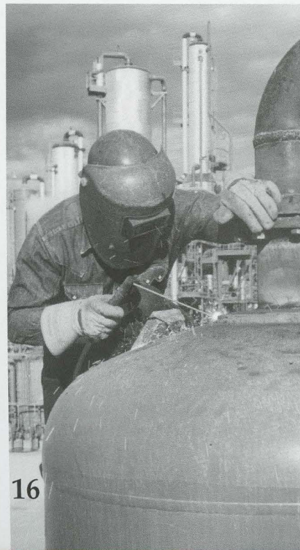
Installation of Liquid Separator for Ammonia Plant, 1961
