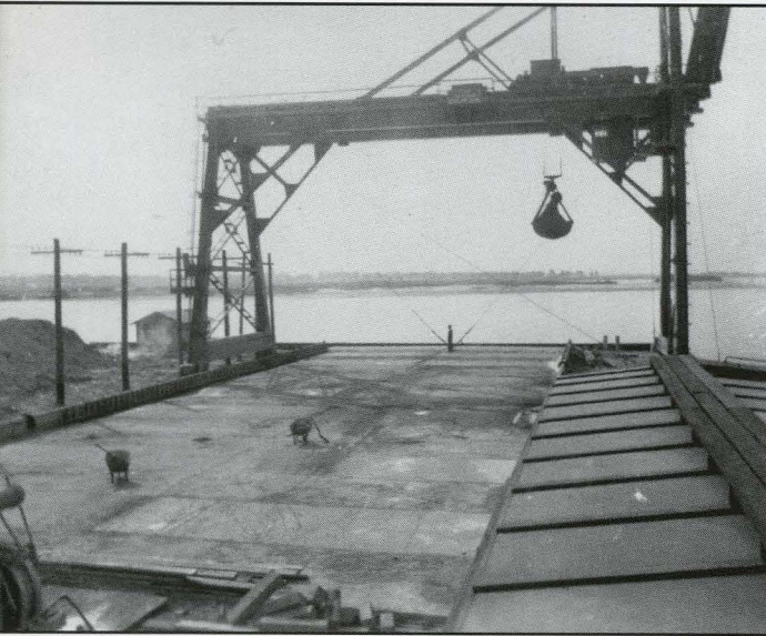
Concrete floor at docks, November 6, 1930
