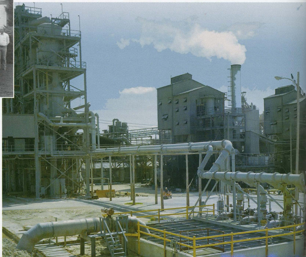
These Prayon Plant Swenson Evaporators (far right) were part of the Pollution Abatement Program improvements.
